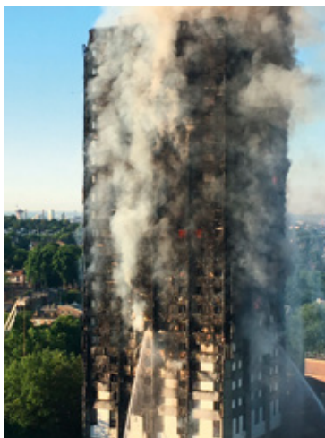
Grenfell Tower - Londra
